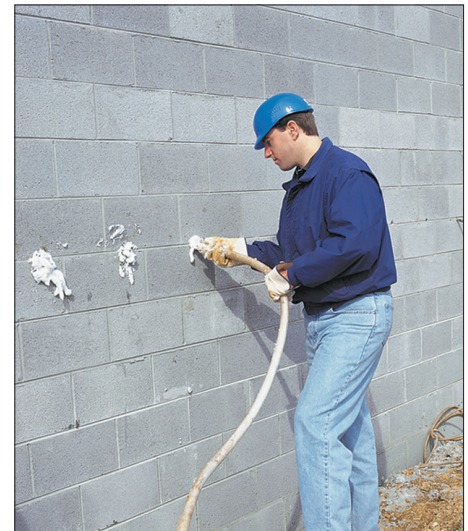
Typical installation technique for Polymaster R-501
