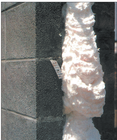
Polymaster R-501 applied in wythe cavity
